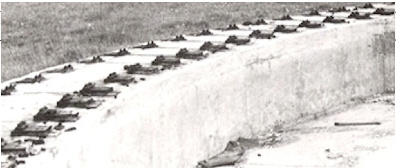
Fig. 14: A block on the mounting plate on the inside end of all ties of Be-10 at Hundborg (source: Hundborg Lokalhistoriske Arkiv ; used with permission)
