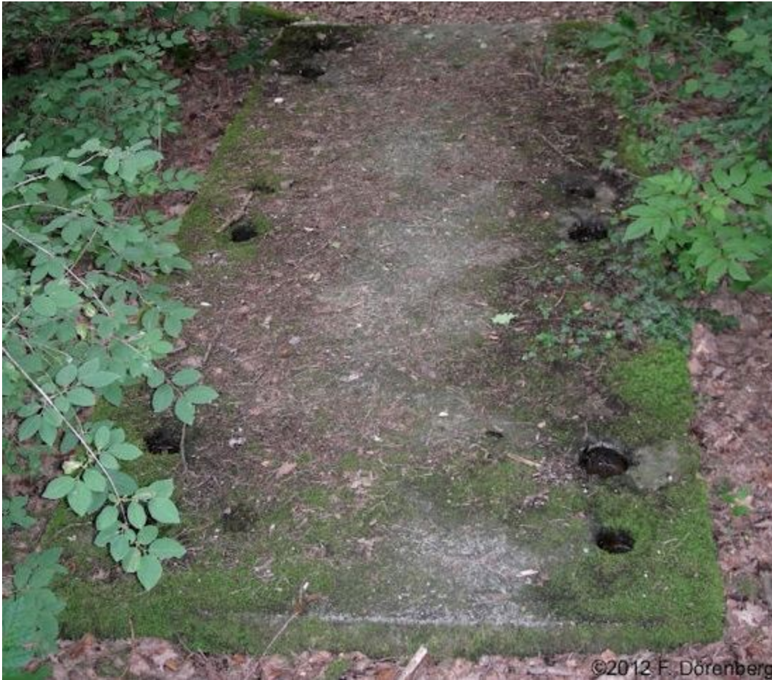
Fig. 178: A concrete slab in the middle of an ancillary building of Be-13 at Aidlingen/Venusberg
