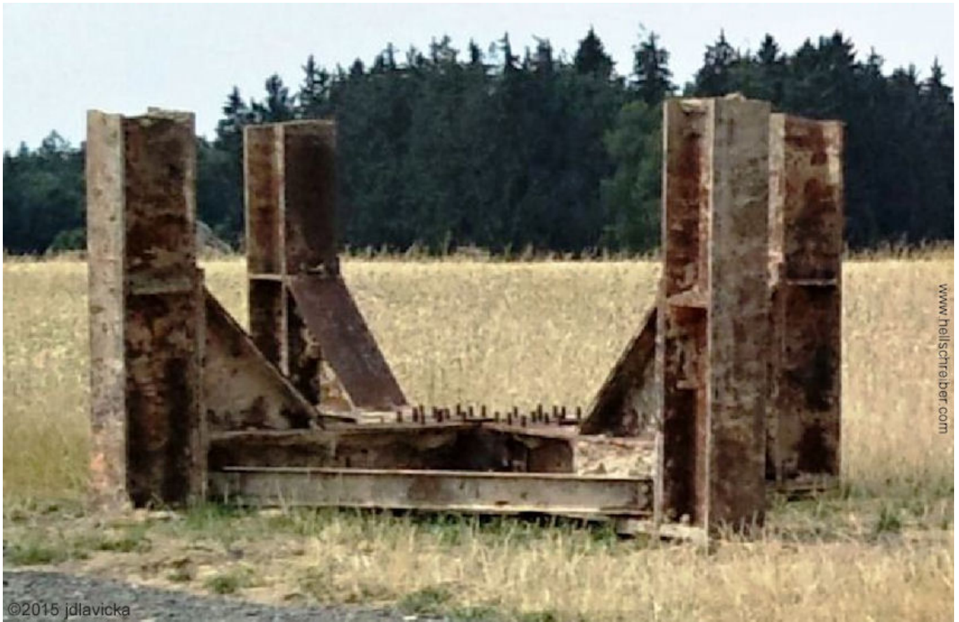
Fig. 45A: The remains of the steel structure of Be-12 , after destruction of the building in 2015
