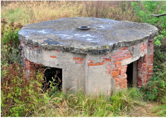
Fig. 47: The round building with the raceway of a large ball bearing in the middle of the roof
