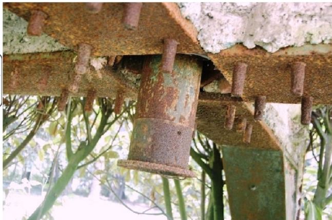
Fig. 48: Tubular shaft descending through the roof of Be-6 at Marlemont and Be-10 at Hundborg
