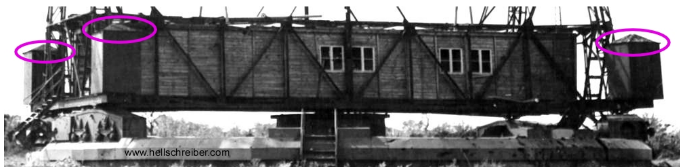
Figure 58: Corner-sheds with a pointed roof (Be-4 at La Pernelle/France)
