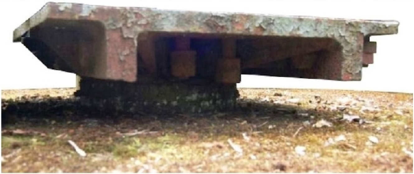
Fig. 49: small turntable on top of the shaft (Be-6 at Marlemont; note the large mounting bolts inserted into the turntable from below)
