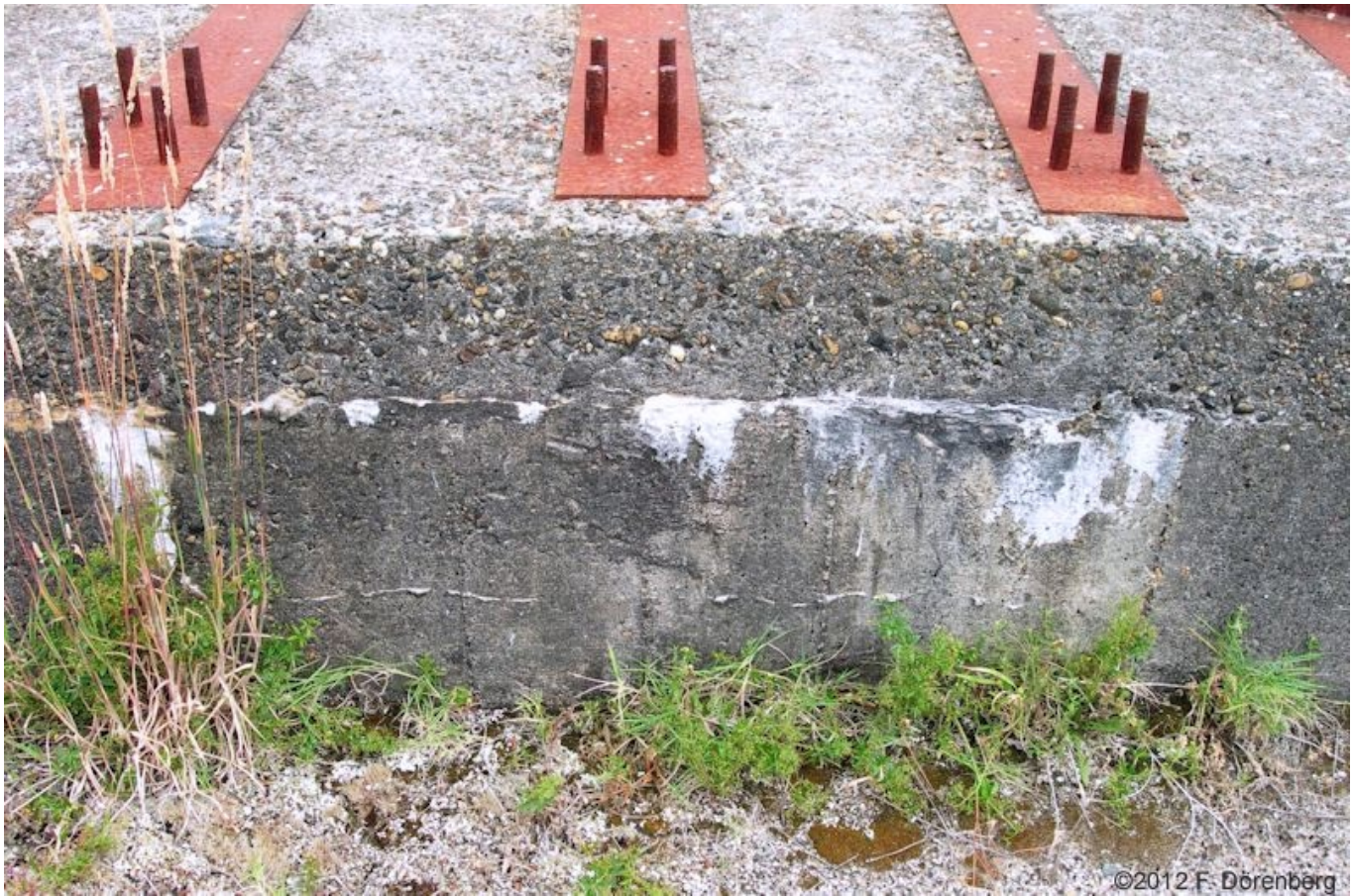
Fig. 11: Top layer of concrete, with embedded I-beam rail-tie at Arcachon
