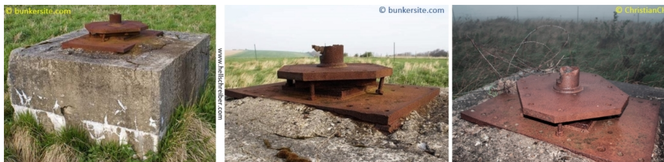
Fig. 46B: The concrete central support block with pivot of "Small Knickebein" station Kn-13
