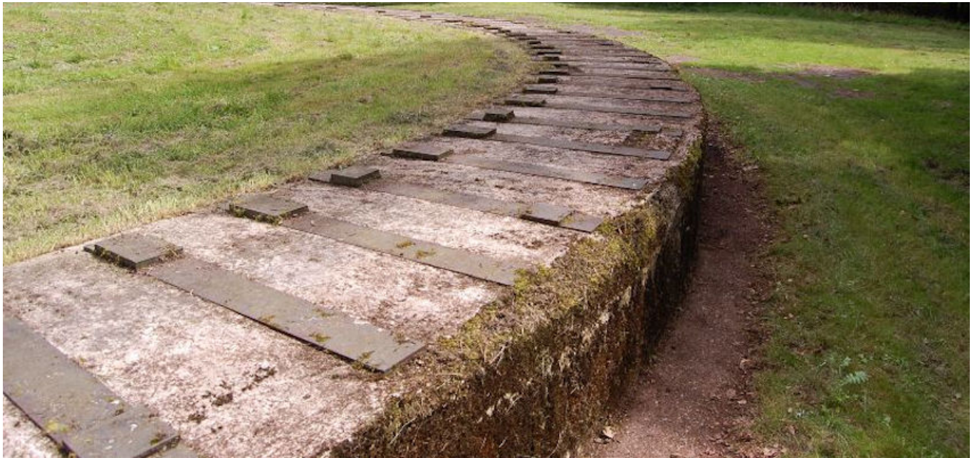
Fig. 13: A block on the inside end of all ties of Be-6 at Marlemont (source: unknown)
