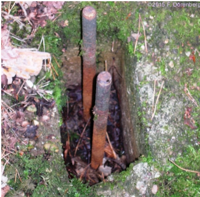
Fig. 9: Pairs of threaded rods
