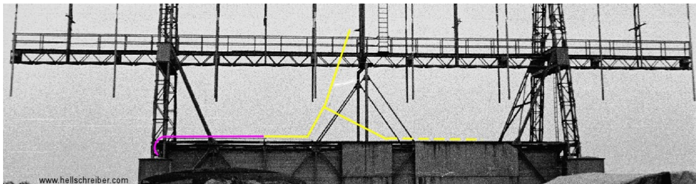
Fig. 123: Routing of the twin-lead cable (pink) and open-wire feedline (yellow) for the bottom dipoles at Bredsted
