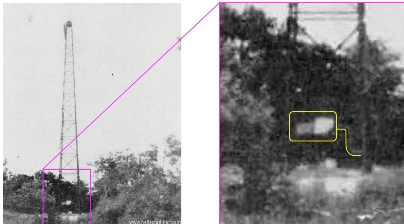
Fig. 184: Monitoring mast - remote-receiver and cable installed at the bottom of the mast (source: ref. 13; probably Be-4 at La Pernelle , based on the other photos in ref. 13)
