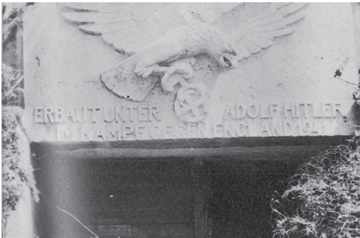
5c. Entrance to the operational dugout of a Knickebein (Kn X on Figure 8 ) erected south of Cherbourg in 1941.
