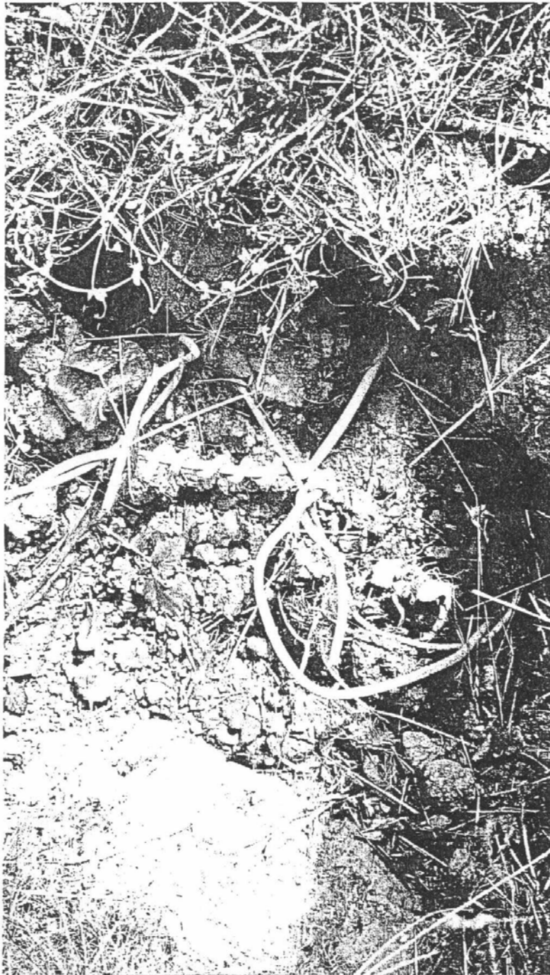
PTB/Fig. 32: #4 ground wires
