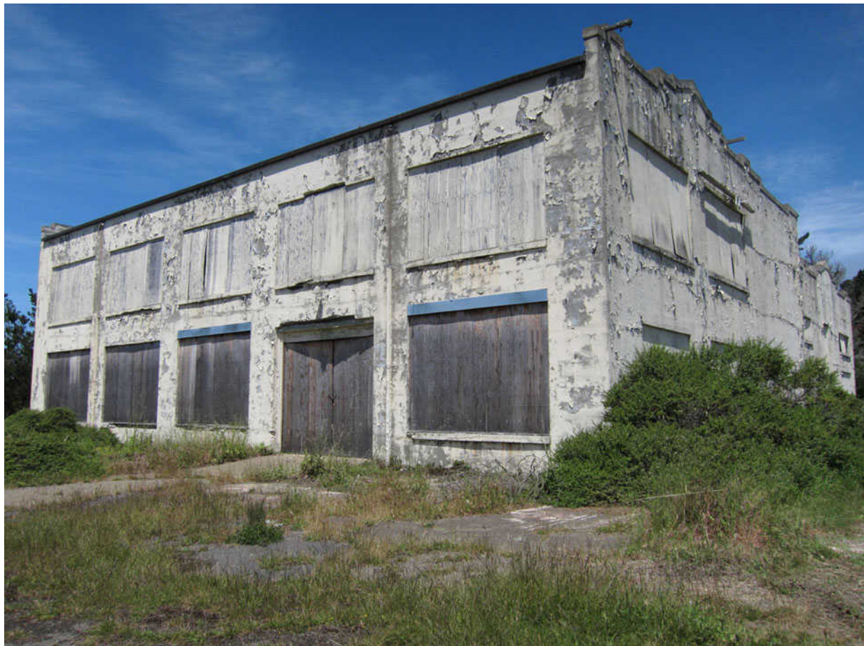
Marconi Power House Building, current condition
