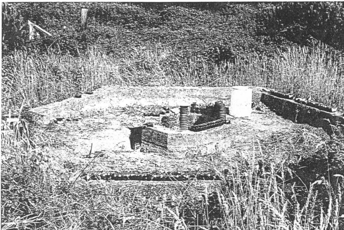
PTB/ Fig UNKNOWN coal shack Foundation
