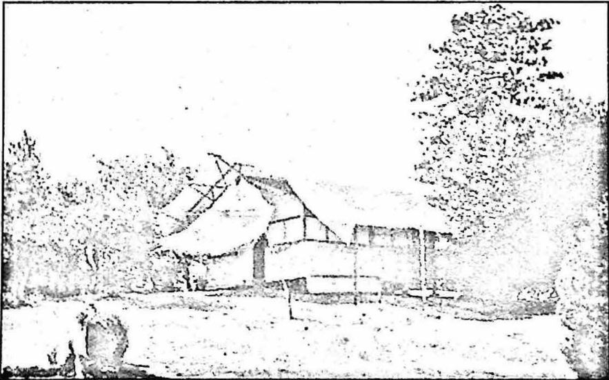
Figure 28. Miller's New Interferometer House, Mount Wilson, 1924, Grass-Covered Knoll. Above, the house with canvas-covered windows all around, and insulating beaver-board walls (wood fiber composite). Below, the same house is fitted with a tent cover over the roof and walls to further stabilize temperatures.
