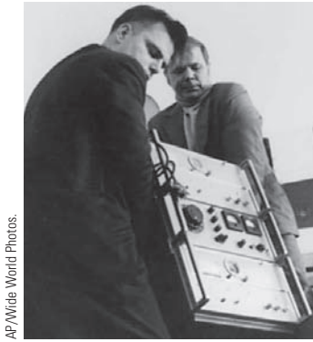
Figure 2.19 Joseph Hafele and Richard Keating are shown unloading one of their atomic clocks and the associated electronics from an airplane in Tel Aviv, Israel, during a stopover in November 1971 on their round-the-world trip to test special relativity.
